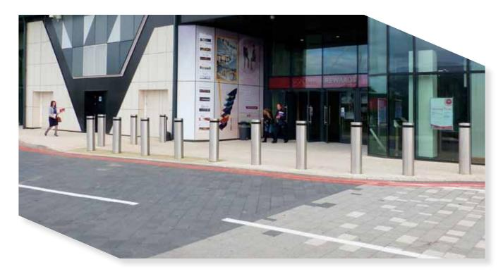
The Terra Venus Bollards has been successfully impact tested to the British PAS 68 specification stopping 7.5t @ 30mph (48kph). Polyester Powder Coated as standard, with a range of sleeves available including stainless steel finishes.
